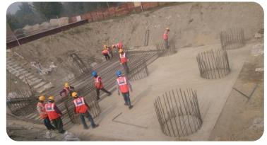
construction drawings and got approved from client. The Reinforcement shall be cut using cutting machines or manually as required and bent at Rebar yard. The bars touching up may be done using wire brush if required to ensure that the bars are free from dust & rust. The rebar shall be transported to location in trailer / truck to the location or manually depending upon the lead.
