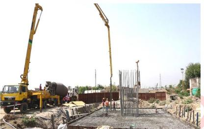
manner to avoid cold joints and compacted by suitable vibration. Shear keys should be located in proper location for pier areas.
