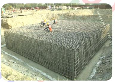
& laps shall be jointly measured after completion of cage placing. Chairs and spacers shall be provided as approved by client. After getting the clearance; balance shuttering work will be taken up. Pier rebar shall be hold in position rigidly to prevent it from buckling.
