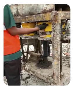
The mixing Motor should be 350 W, 400 rpm electric hand drilling machine or proper mixing table as recommended. The speed of 400 rpm should not be exceeded because higher revolutions will entrap air in the mix.
