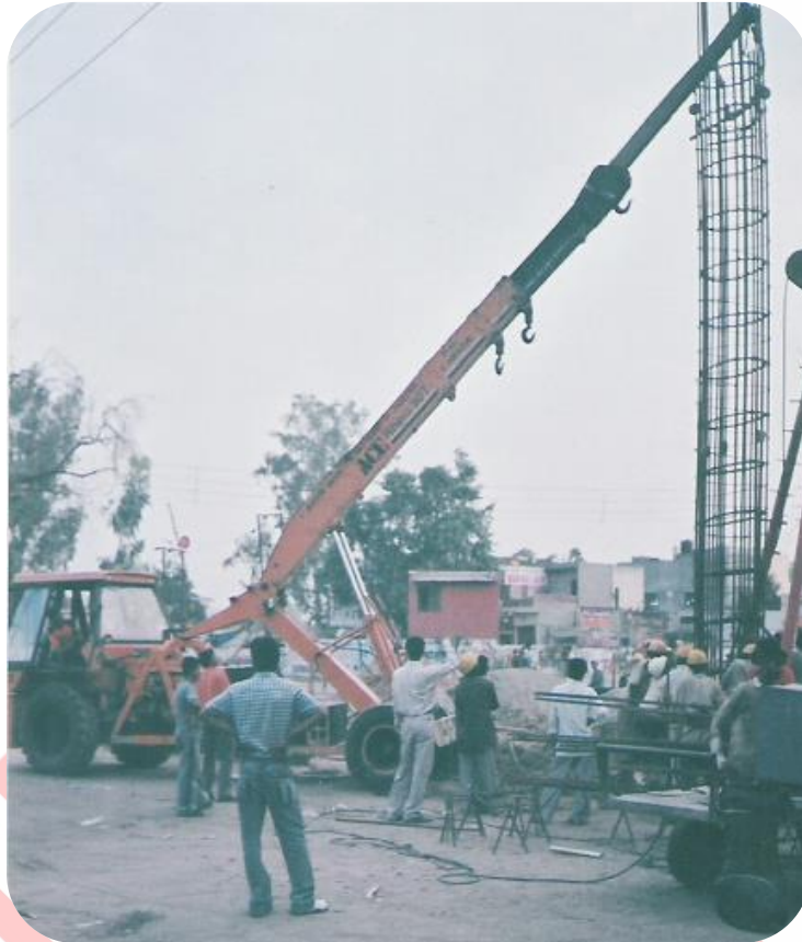
Installation of reinforcement cage into the pile hole
