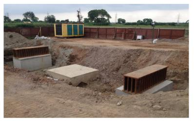
cast with a suitable pile head as detailed in drawing. Suitable structural arrangement shall be made to facilitate fixing of magnetic stand and deflecto meter for measuring the settlement of pile.
